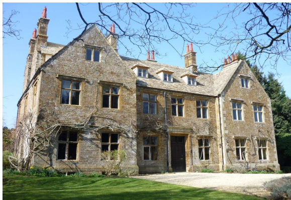
The Grange Adderbury, recently restored
