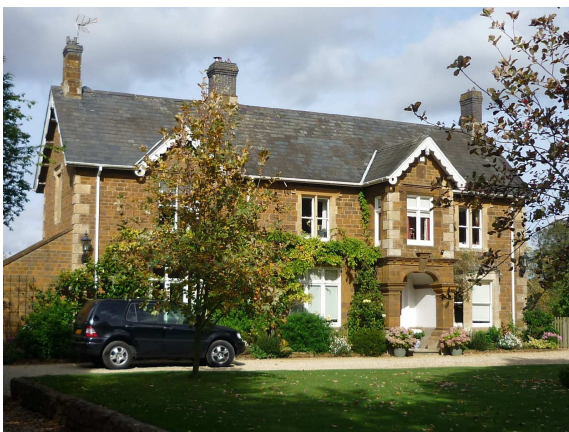
Holmby House, Sibford Ferris, nineteenth century gentleman's villa, an undesignated heritage asset
