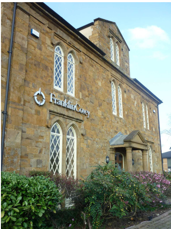
We served a Repairs Notice on Grimsbury Manor, which is now beautifully restored
