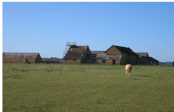
Combe Hill Farm, Milton, an Inclosures farm built in the mid 18th century with all out buildings in tact and now curtilage listed
