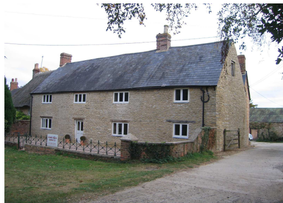
Montague Farm, Hethe (grade II), after restoration
